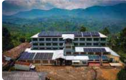
Solar Power Project – Stockholm Tea Factory
